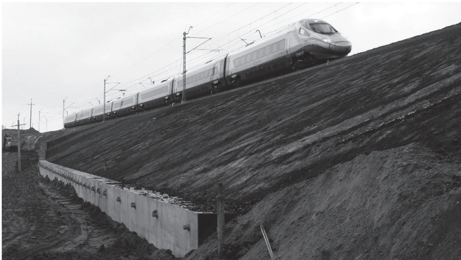
Fig. 10: Rebuild embankment on landslide side
